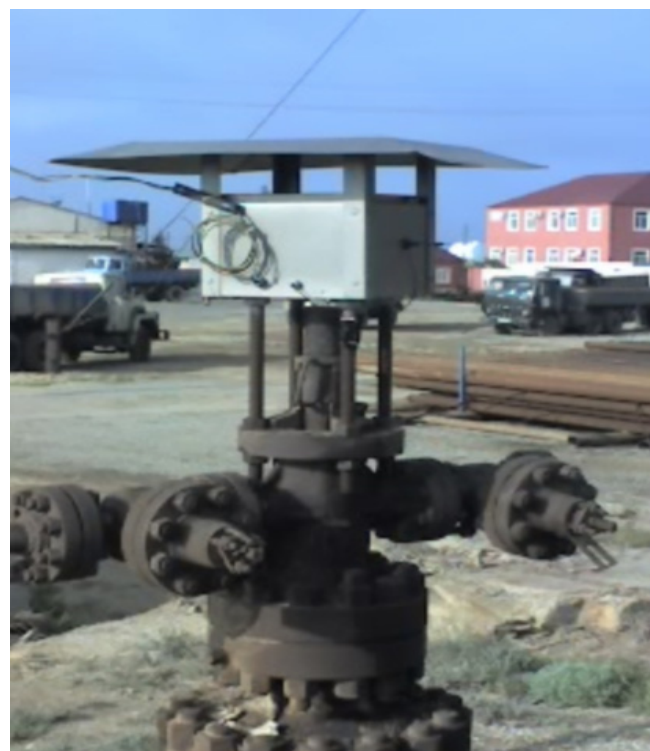
Figure 2b. Appearance of the station after installation
