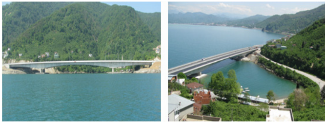
Figure 1. Some views of Gulburnu Highway Bridge.
