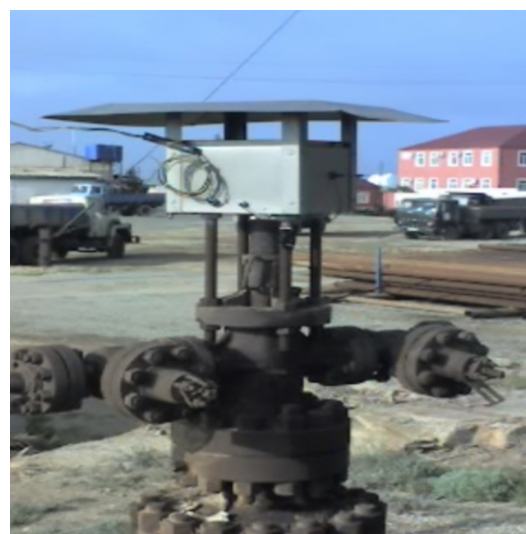
Figure 2. Appearance of the station after installation
